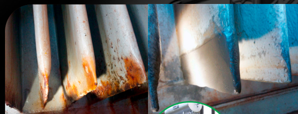
Oil leak repair with MAX 5611 on a power transformer radiator.
