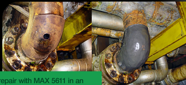
Repair of an oil leak in an offshore pipe weld seam using MAX 5611.
